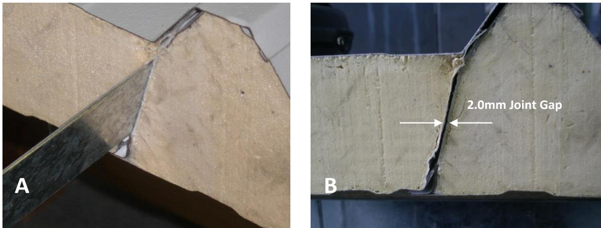
*Figure 24: A) Steel packing piece used for 2.0mm joint gap, B) Resulting 2.0mm joint gap formed between the panels after assembly to the support structure*
