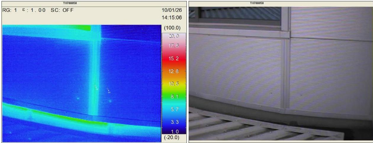
Figure 48: The same planar joint showing thermal losses along the length of the joint, indicating missing or incorrectly installed insulation
