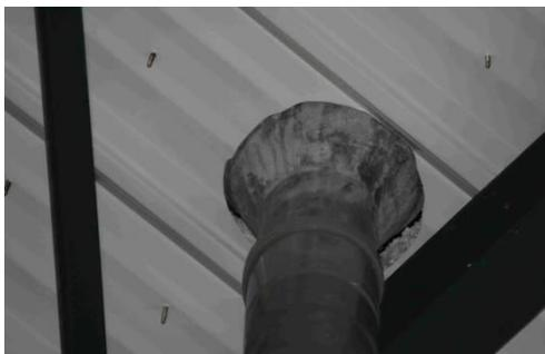
Figure 7: Drainage openings in roofs: Thermal bridge + air tightness gap
