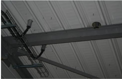
*Figure 8: Openings in roof; electrical wiring and small structural supports*
