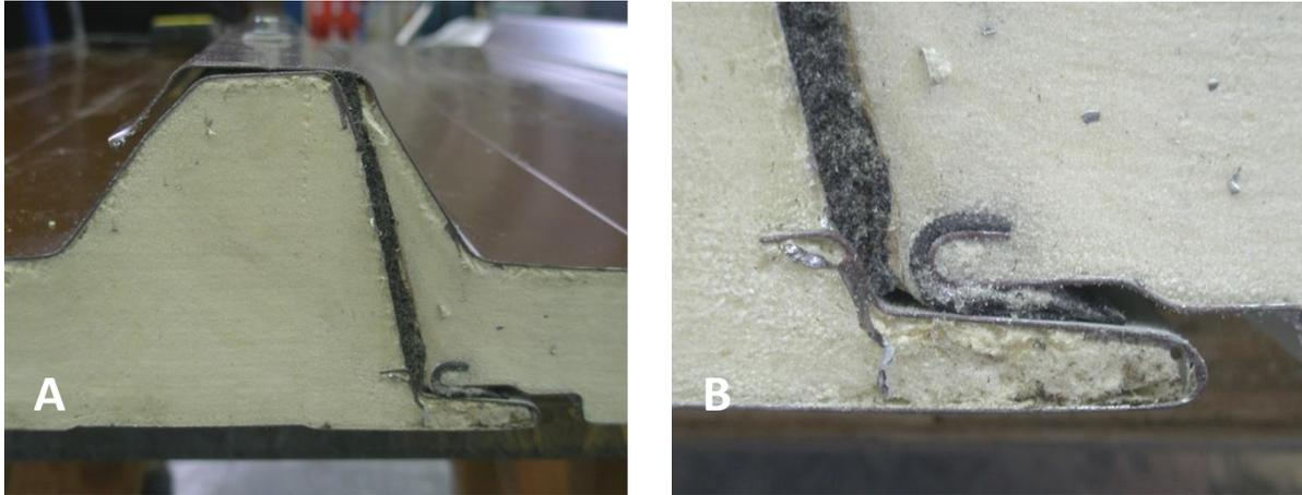
Figure 25: A) The FischerTHERM composite panel side lap joint when assembled, B) Close up picture of the EPDM gasket seal
