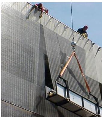
Figure 59: Stainless steel meshes used as solar shading systems
