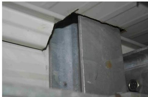
*Figure 9: Structural penetration in the envelope*
