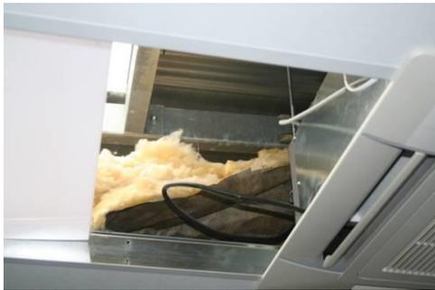
*Figure 19: Unfinished interface at sky dome arrangement*
