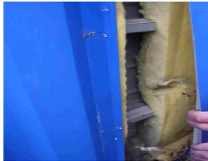
*Figure 20: Missing path of mineral wool*
