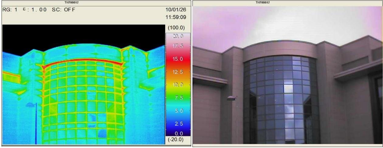
Figure 42: Heat rising from the built-up system which divides the windows causing a stack/chimney effect, contributing to the accumulation at the top of built-up feature
