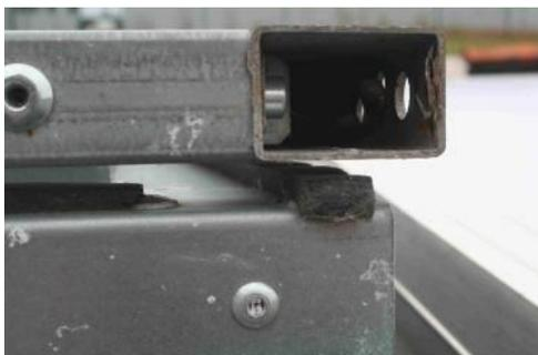
*Figure 10: Unefficient skydome joints*
