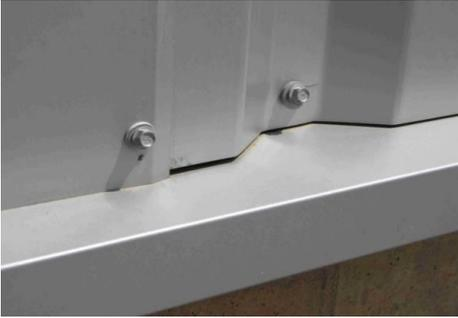
Moisture and corrosion at joint showing air penetration and condensation
